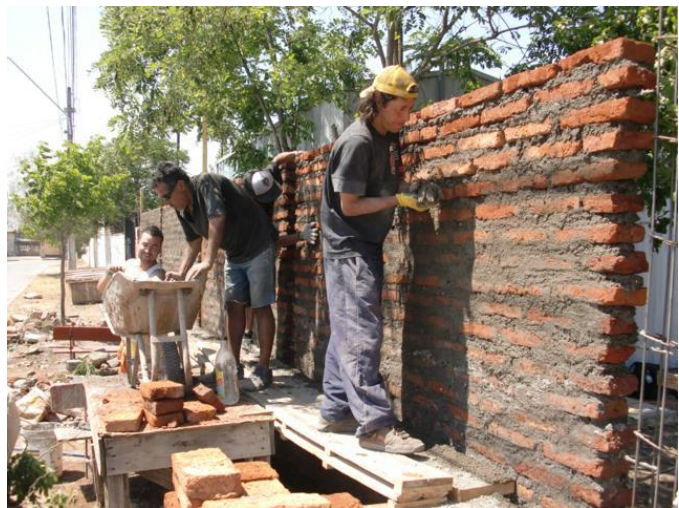
Reconstructing clinic property walls that were destroyed during the earthquake.
